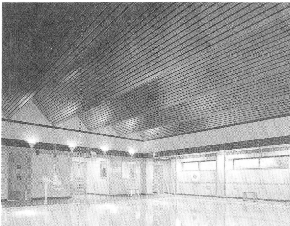
Figure 6-3 Brooks Army Medical Center, San Antonio, Texas, features PLANAR®, an Interfinish™ brand product from Chicago Metallic. (Photo courtesy of Interfinish brand products of Chicago Metallic.)
