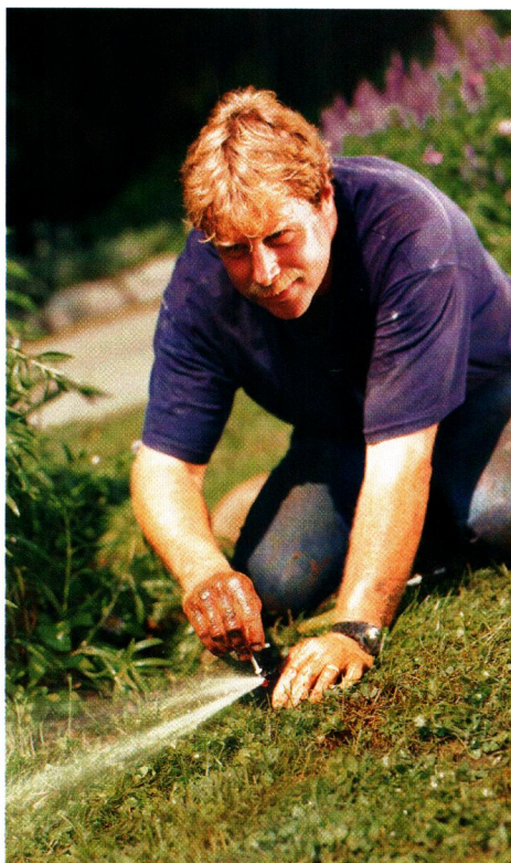
At the end of the project, sprinkler heads get a final adjustment to ensure they're covering intended areas.
